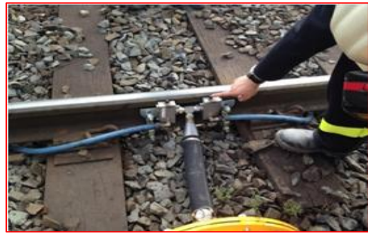
This picture shows the Rail Grease Unit.
