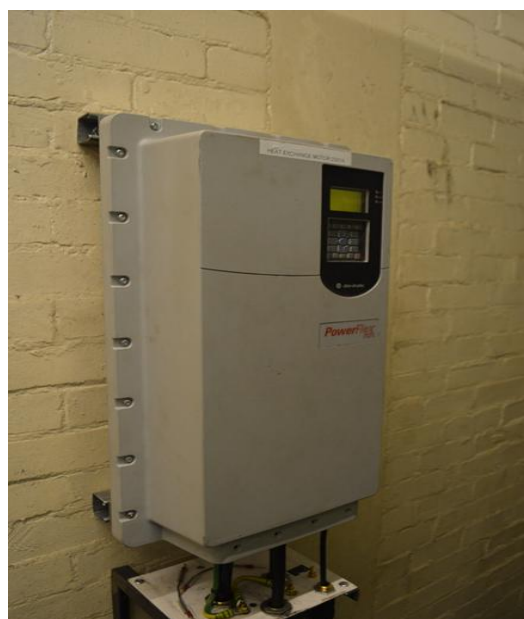
This picture shows the VSD on Circuit 1
